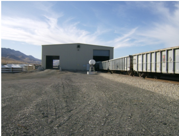
The MHF-operated transload facility at a Nevada mine site.
