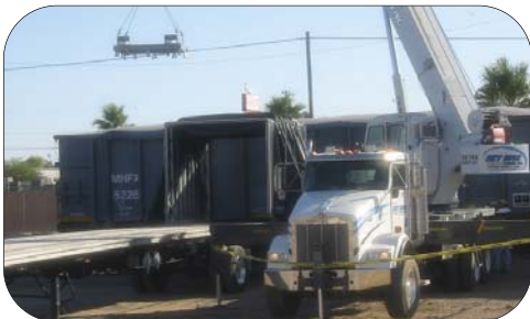
Railcar offloading operations at Parker, Arizona Transload Facility.
